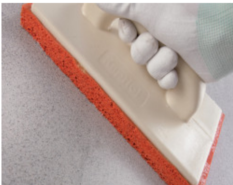
Finishing off the surface of the smoothing and levelling layer with a sponge float
