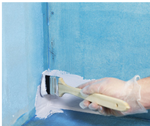
Mapei nurgatihendi IC/EC paigaldamine Mapegum WPS-i abil
